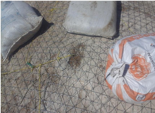
Sand bags over wire mesh
