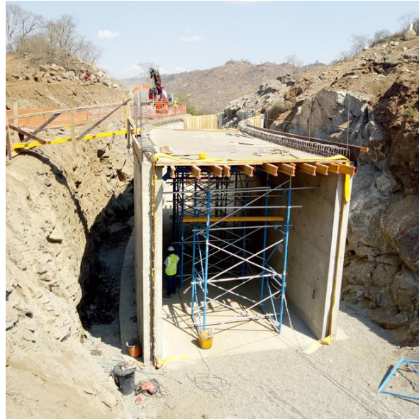
Tedzani 4 HEP Project Tunnel Construction
