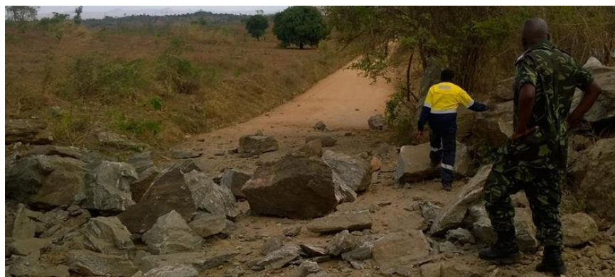
HEMA Construction Company – Mwanza – Tsangano Border Road Construction
