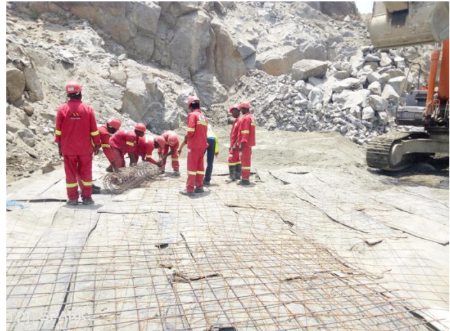
Wire mesh over Rubber sheet then sand will be on top
