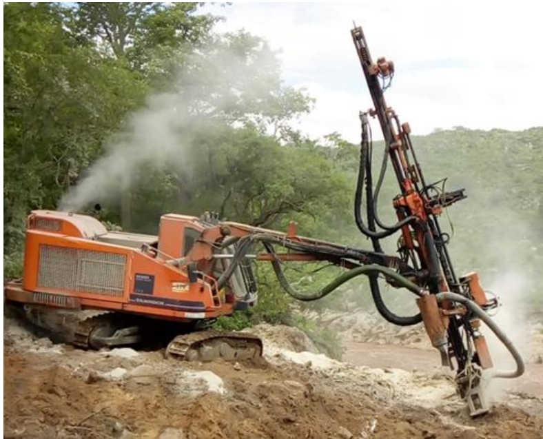
Hydraulic Rock Drilling Machine (Airtrack) at work. Photo MS 2019
