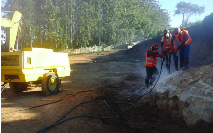
Hand held Rock Drilling Machine at work
